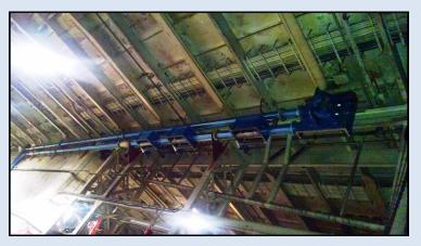
Once the conveyor tubes are up to the overhead ceiling of the car deck there is more room but the conveyor is high in the air which brings its own set of installation challenges.
